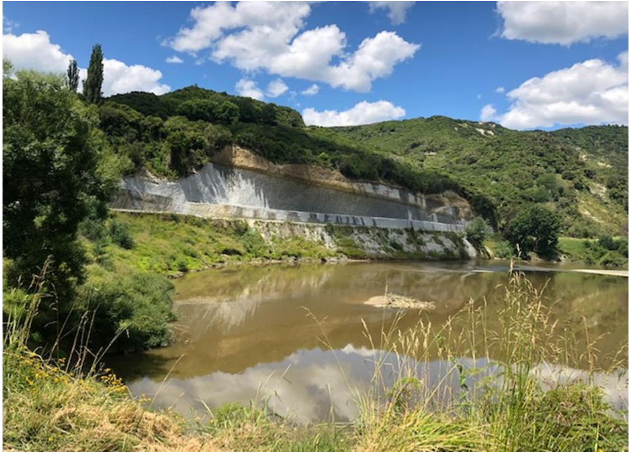
Photo: Taken standing on the August 2018 Jerusalem dropout, looking over to the June 2015 completed repair
